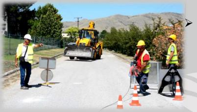
Arrival of contractor's JCB excavator, in order to carry out necessary excavations, cutting and topping of the service line in order to be able to repair the station.
