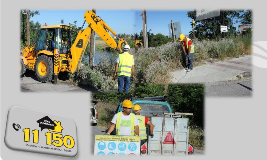
➤ Staff of the contractor company arrives at the incident venue to excavate, cut and tighten the pipeline around the bridge so as to secure the part of the pipeline.
